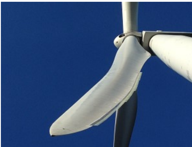
Fig. 1: LNTEs on the wind turbine rotor blade
