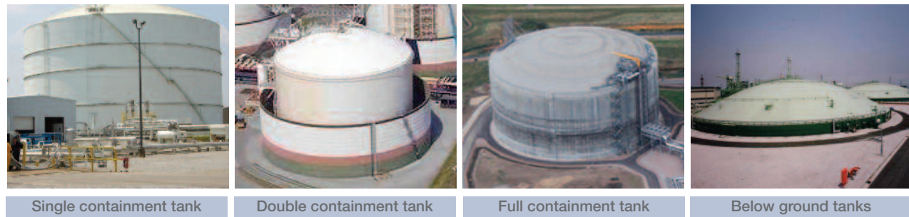
Figure 2.4 Four types of commercial LNG storage tank
