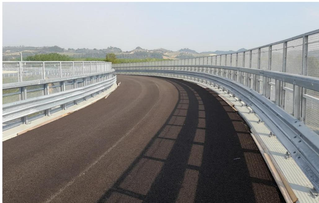
**FIGURA 2-21 RAMPA DI INGRESSO ALBA OVEST-CUNEO – SICURVIA BORDO PONTE, INTEGRATO CON RETE ANTISCAVALCO**
