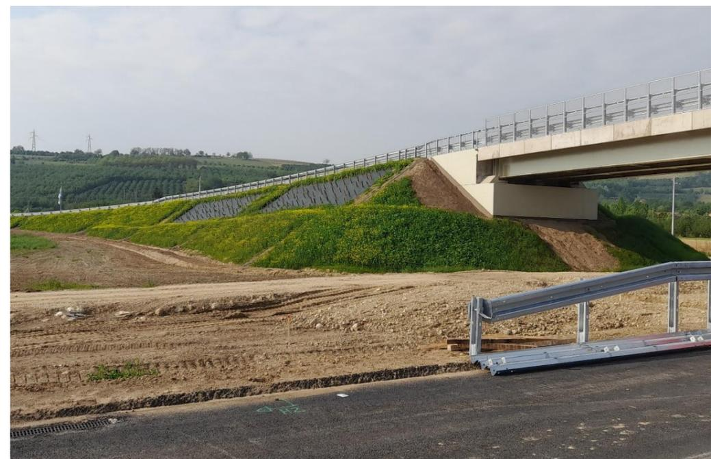
**FIGURA 2-16 CAVALCAVIA STRADA CAMPESTRE ALLA PROGR. 5+915.15 – PARTICOLARE CORPO SPALLA AMMORSATA NEL RILEVATO DI APPROCCIO ALL'OPERA**
