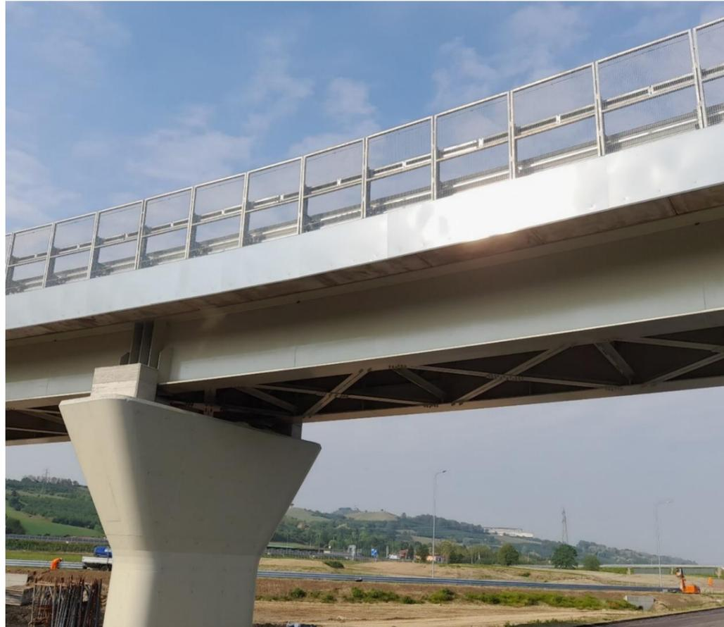
**FIGURA 2-20 RAMPA DI USCITA ASTI-ALBA OVEST – VISTA DELLA RETE ANTISCAVALCO E DELLE VELETTE DI MASCHERAMENTO**
