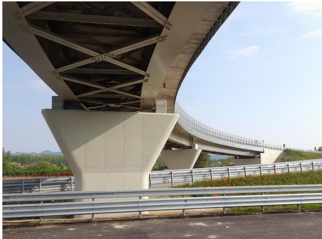
**FIGURA 2-13 RAMPA DI USCITA ASTI-ALBA OVEST – VISTA DELLA PILA E DEL SISTEMA DEGLI APPOGGI E DEGLI ELEMENTI DI RITENUTA ANTISISMICI**
