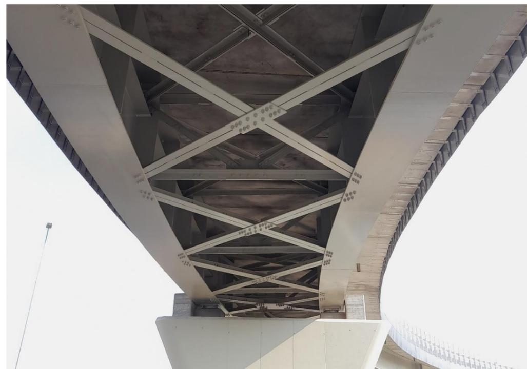
**FIGURA 2-14 RAMPA DI USCITA ASTI-ALBA OVEST – VISTA DI DETTAGLIO DELLA STRUTTURA A TRAVI VERTICALI DELL'IMPALCATO**
