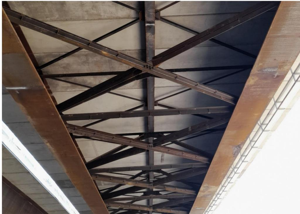
**FIGURA 2-7 PARTICOLARE DELL'IMPALCATO METALLICO A TRAVI INCLINATE E CONTROVENTI**
