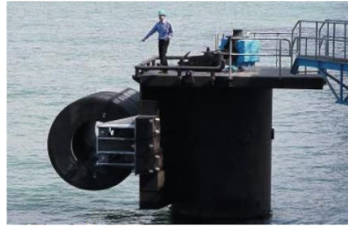
▲ Power Station Coal Berth
