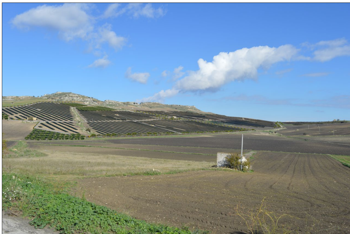
Figura 90 - AD.1 Post operam
