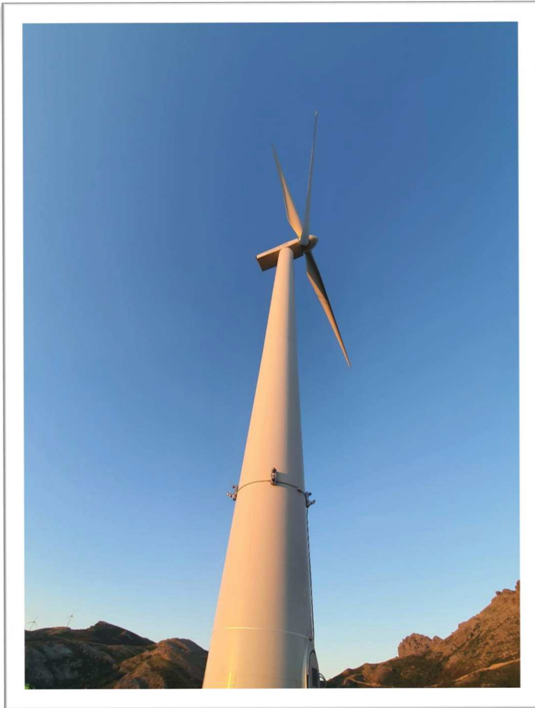
[Outside installation overview – SIEMENS GAMESA}
