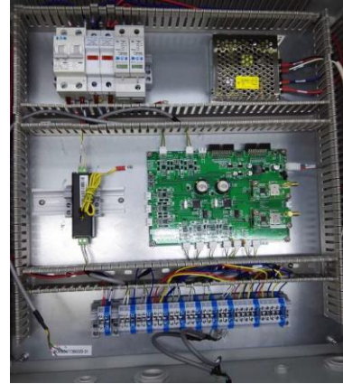
Figure 23, Internal components of the communication box
