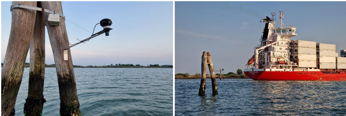
Fig. 2.2 - Ultrasonic tide gauge installed on bricola 121 next to the channel (left) and Louise Borchard ship passage (right).
