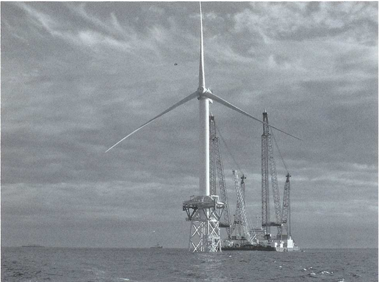
Fig. 1-1. Turbina eolica 5M in montaggio (REpower)
