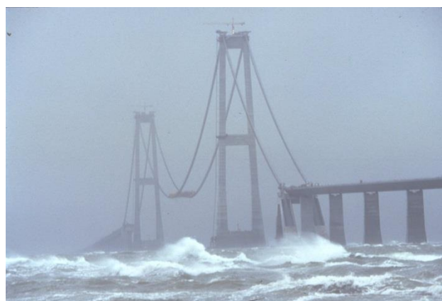
The directional decoupled parametric formulation in MIKE 21 SW is used extensively for calculation of the wave transformation from deep-water to the shoreline and for wind-wave generation in local areas
