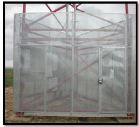
Figure 5. Anti-climb fence
