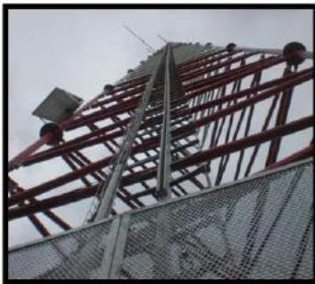
Figure 6. Fall arrest system
