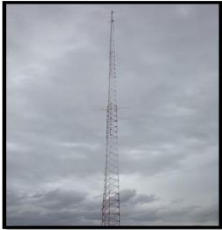
Figure 1. Met Mast Structure
