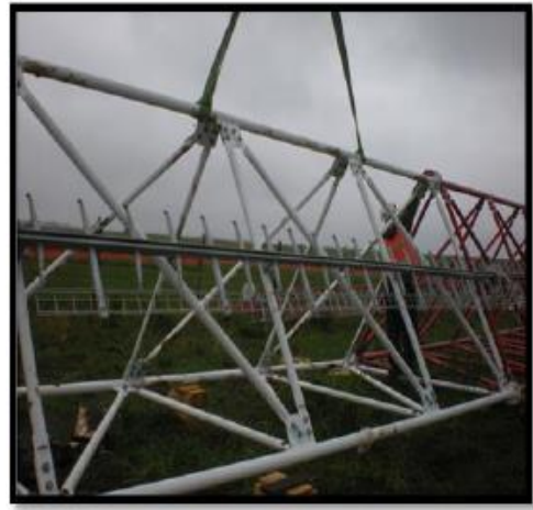
Figure 2. Met Mast Structure
