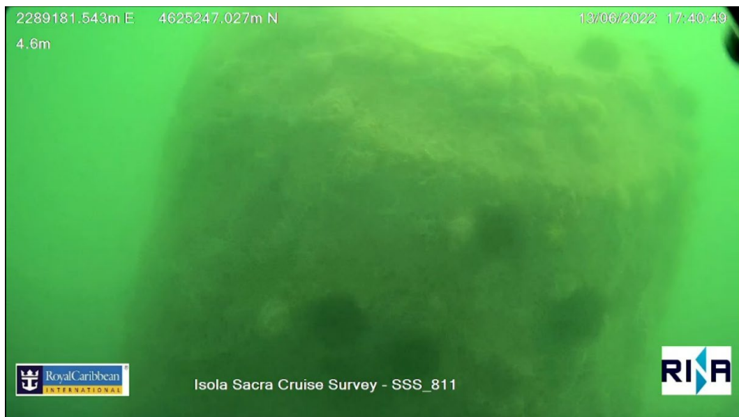
Figure 4.27: TA 811 pole with concretions (Echinoidea and algae specimens)
