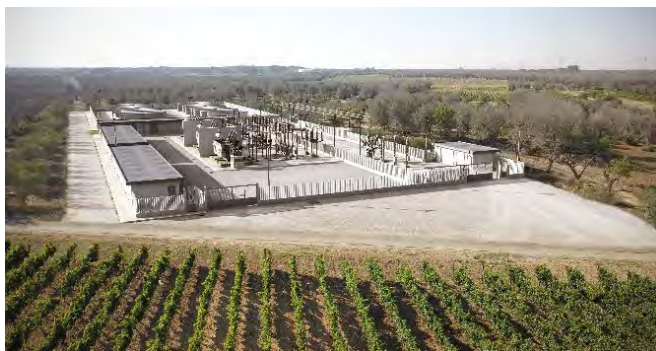
Area cabina post operam
