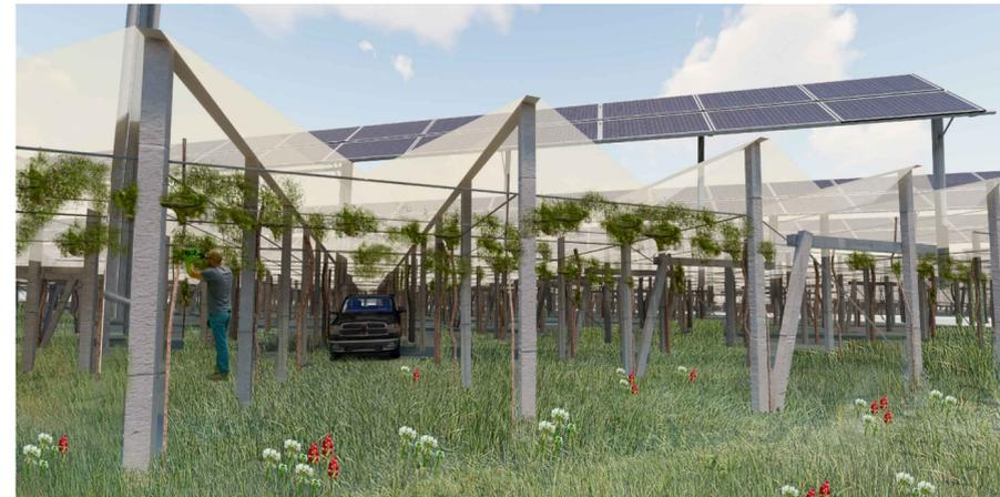
STRUTTURE FOTOVOLTAICHE INTEGRATE AL VIGNETO A TENDONE E AL PRATO FORAGGERO
