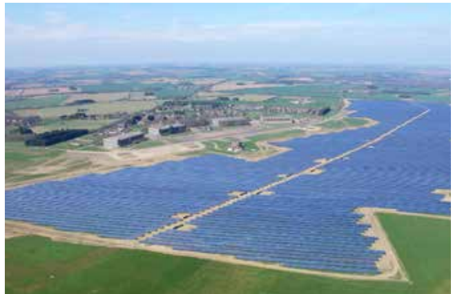
UNITED KINGDOM West Raynham, 44 MW HEC PLUS
