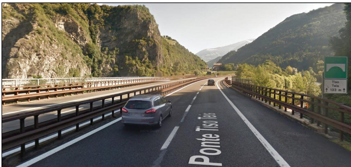
Fig. 1 – Street view del ponte autostradale Tiso – Google Earth
