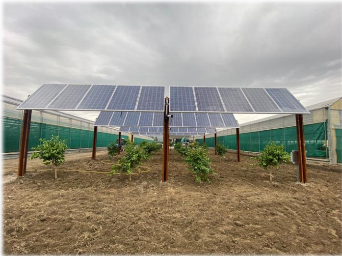
Valmont Solar TRJ tracker supporting medium size trees in the south of Italy
