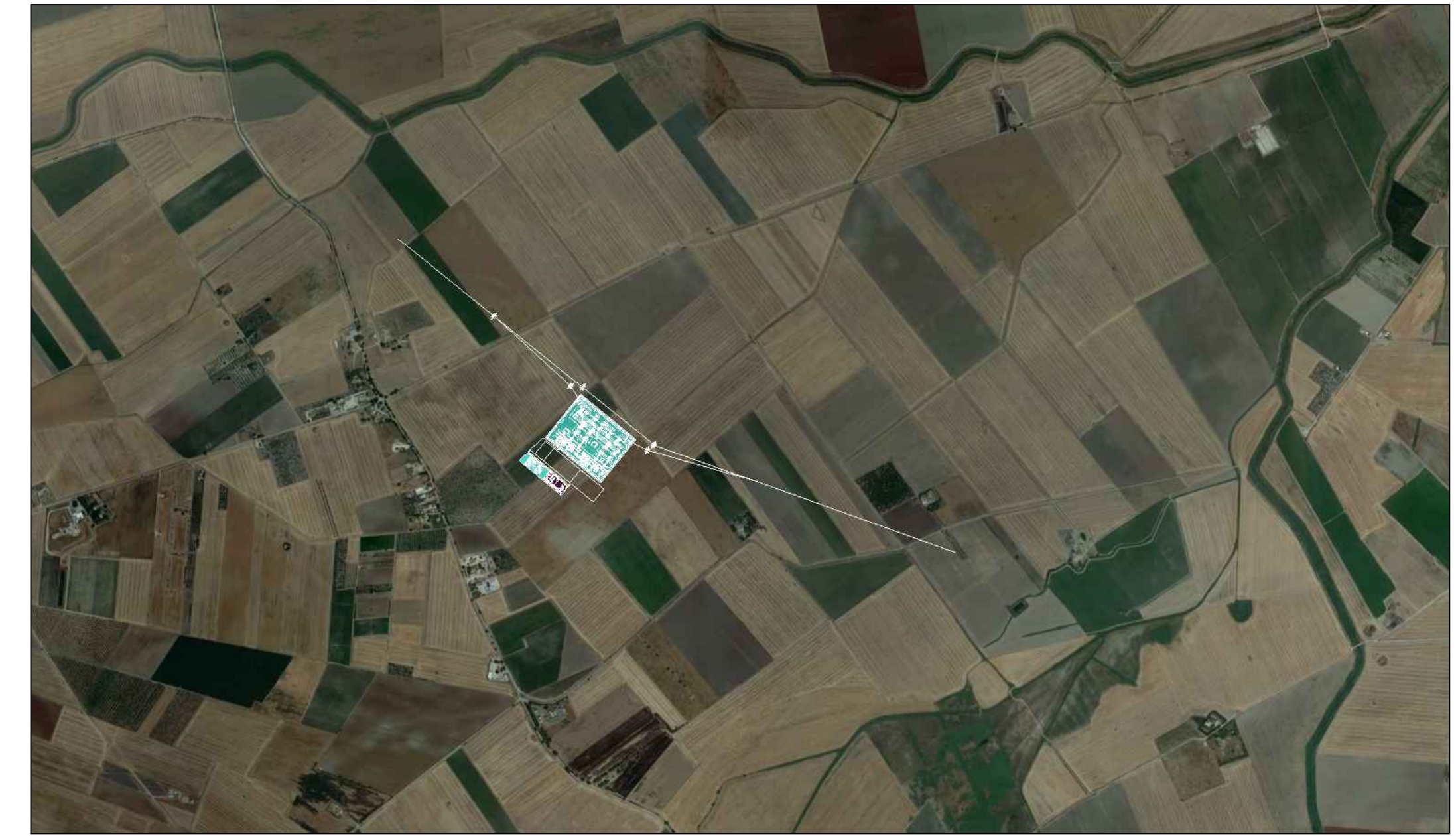
Ortofoto area vasta - post operam
