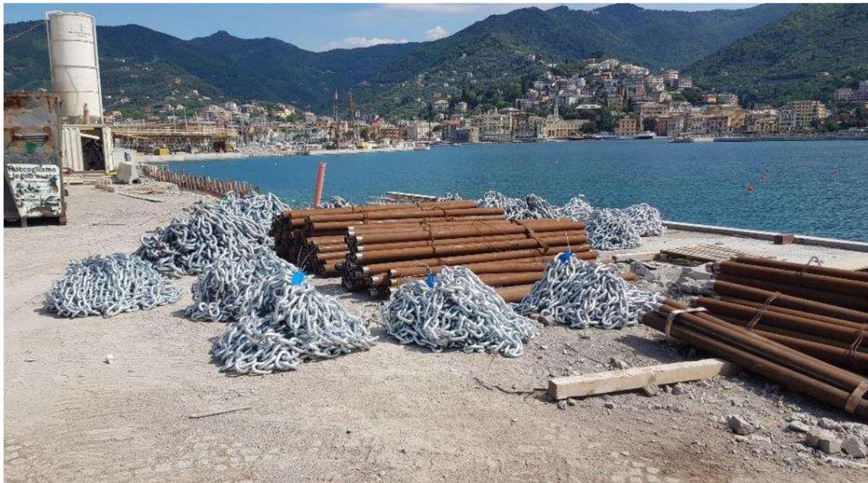
*Foto 19: 08.05.2023 – catenarie ormeggio e tubi jet grouting*
