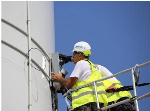
External fixed backplate, wire ropes and mounted system
