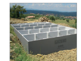
underground water retention basin
