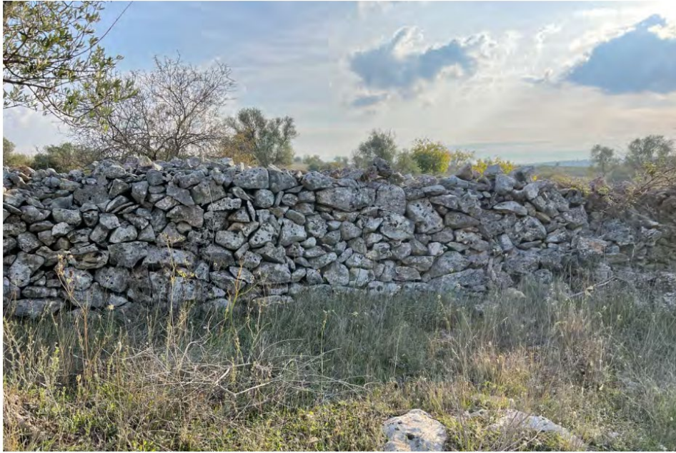
Figure 10: Muretto a secco
