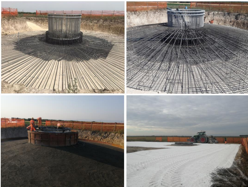
Figura 2—11 – Principali fasi posa in opera plinto
