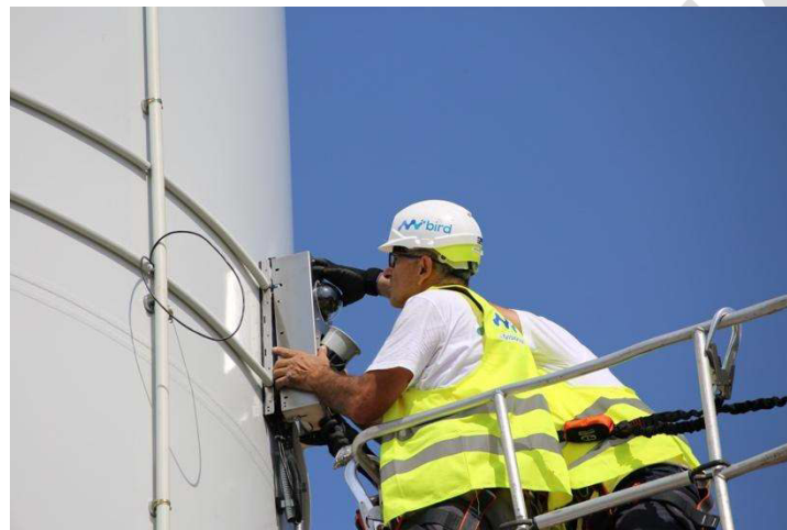
External fixed backplate, wire ropes and mounted system
