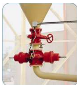
Figure 8.16 Scarico fanghi
