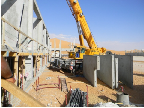
Picture 3: Vertical prefabricate structure Installation
