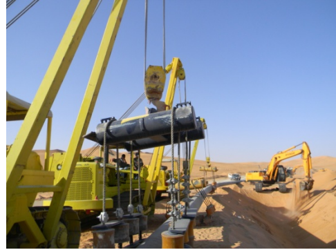
Picture 4: Horizontal prefabricate structure Installation
