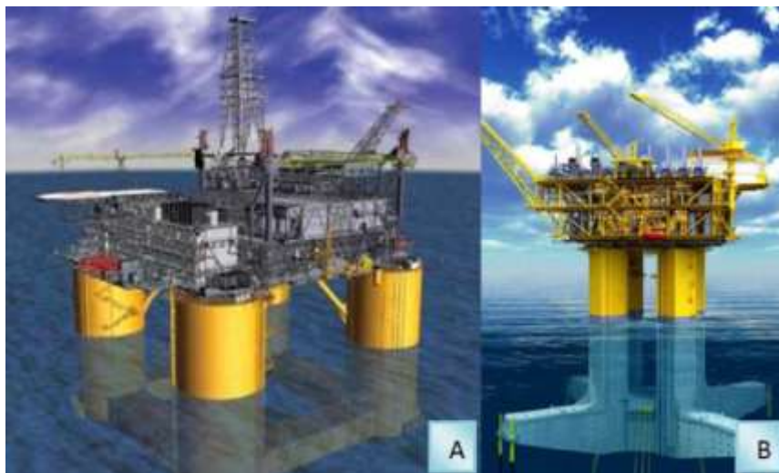
Figure 1.8 Tension leg platforms moored to the seabed (Sources: image on the left ( http://www.offshore-mag.com/articles/print/volume-73/issue-01/gulf-of-mexico/shells-mars-b-develop-begins-take-shape.html ); image on the right ( https://www.rigzone.com/training/insight.asp?insight_id=305&c_id=12 ))
