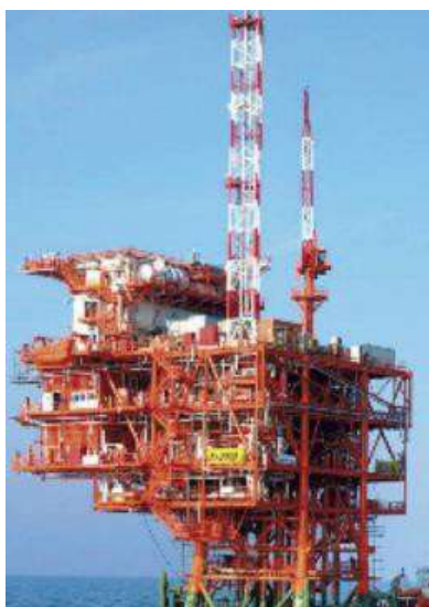
Figure 1.5 Steel frame (jacket) platform resting on the seabed (Source: http://www.ina.hr/UserDocsImages/Ina_casopis/zima09-10/44-45%20annamaria.pdf )
